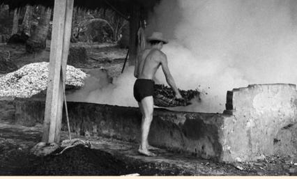
A lime kiln at Kampong Mata Ikan, 1967. Seashells (white pile on the left), which are made of calcium carbonate, are heated to approximately 900 degrees Celsius to produce calcium oxide, also known as quicklime. The man is using a woven rattan pungki or pengki (畚箕) (a shallow basket) to deposit what looks to be charcoal – fuel for the kiln – into an open pit. Photo by Hor Kwok Kin. Retrieved from Photonico.
